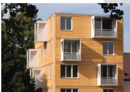
8 City of Wood Bad Aibling
